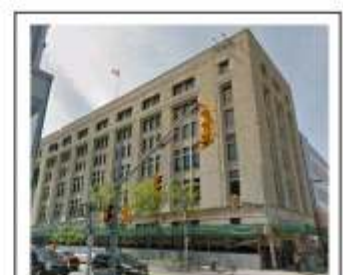
Paul Martin Bldg Windsor
