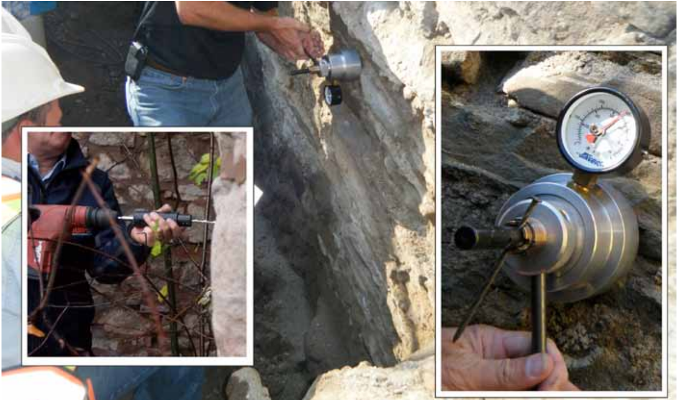
Figure 6. Installing and testing stainless steel helical masonry ties.
