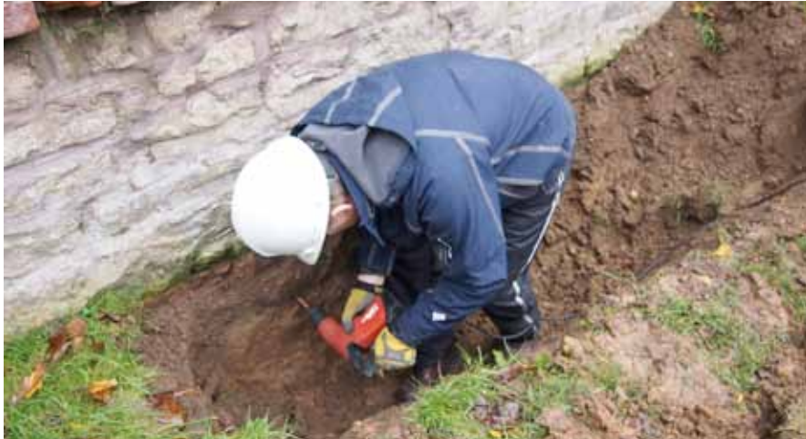
Figure 5. Trial drilling within an excavated inspection trench.
