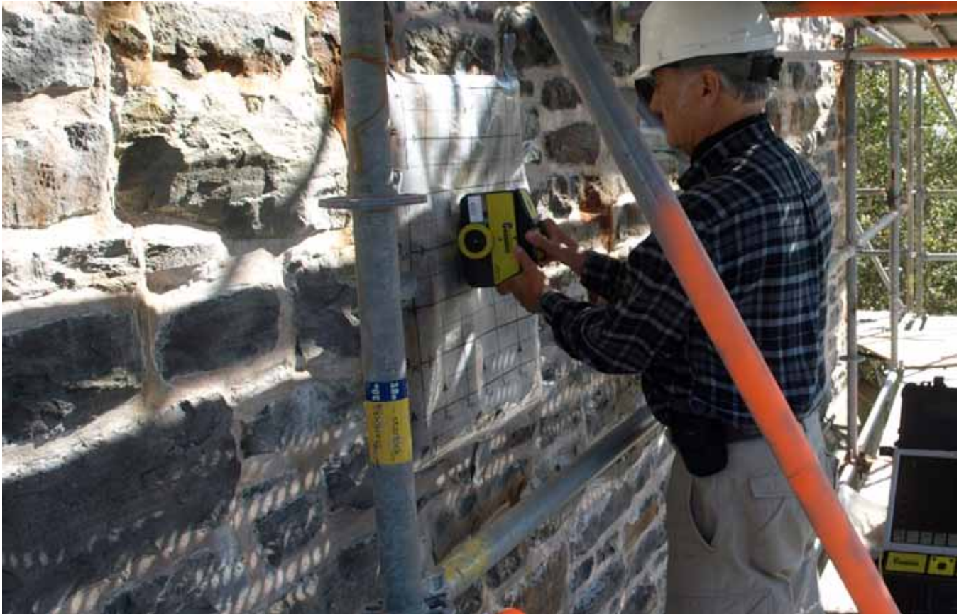
Figures 3. Using ground penetrating radar technique to investigate hidden conditions.
