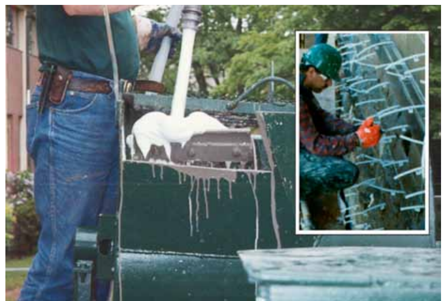
Figure 7. Producing and injecting cellular foamed grout using low pressure grouting techniques.
